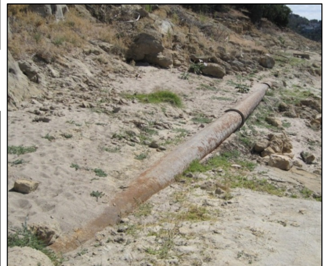
Exposed Interceptor IW-86 on the West Interceptor
