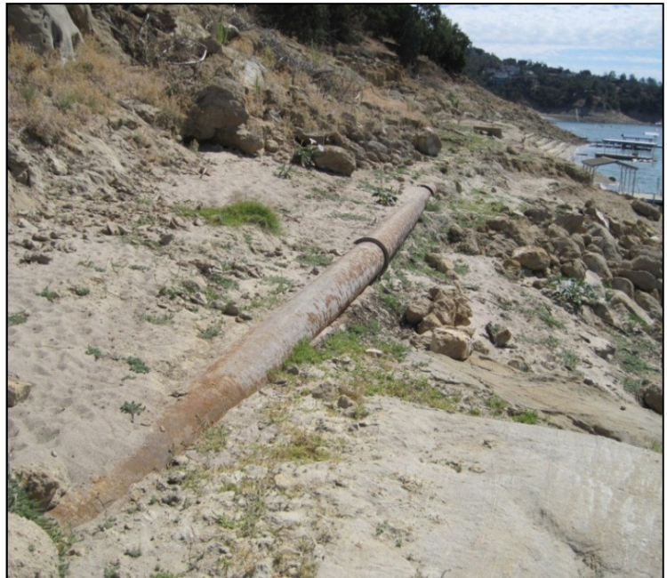
Figure 4.1: Exposed pipe along the West Interceptor between Manholes M86 and M87
