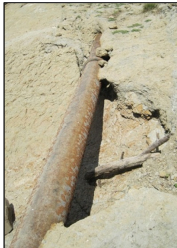
Exposed Interceptor Pipe IE-124 on the East Interceptor
