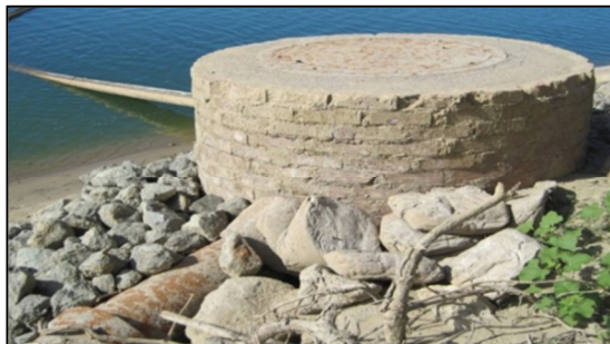
Manhole M93, Exposed Interceptor lower left
