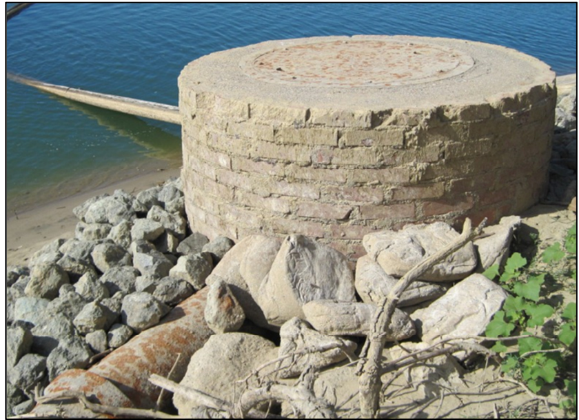
Figure 2.6: Manhole M93, Exposed Interceptor, and Stabilization
