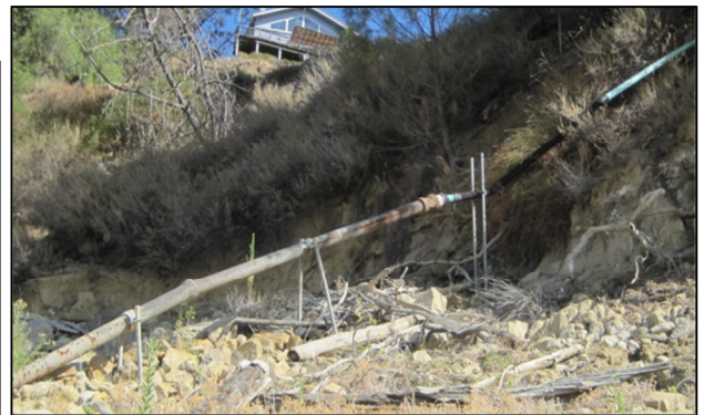
Exposed Lateral Repairs along Eroded Bank
