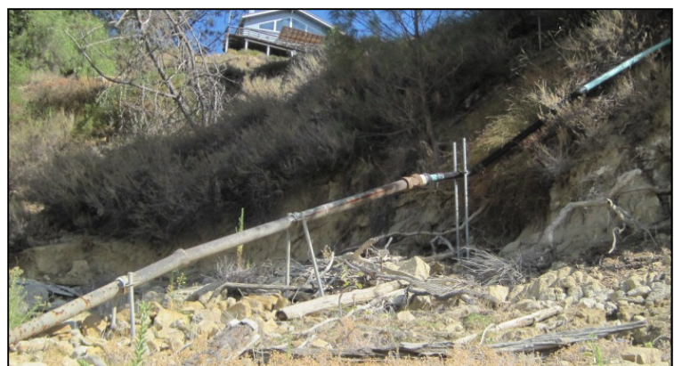
Figure 2.5: Exposed Feeder Composed of Different Materials
