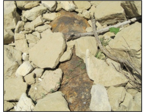
Figure 4.2: Corrosion of Interceptor
