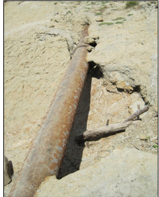
Figure 2.4: Exposed Interceptor Pipe IE-124 on the East Interceptor
