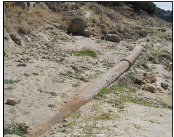
Figure 2.1: Exposed Interceptor IW-86 on the West Interceptor
