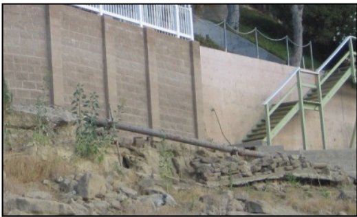
Figure 4.14: Retaining wall built over Feeder F-95
