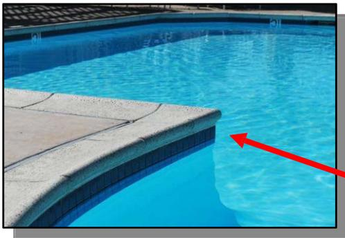
**COPING** around the pool is usually a series of bull-nosed stones that slope away from the pool. This helps keep the pool clean by directing water on the deck away from the pool. Coping also functions as a handhold for bathers and must hang over the pool wall at least 1 inch, but not more than 2 inches. It is not to exceed 2 ½ inches in thickness.
